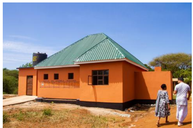
Oldenderet school toilets before and after for 358 students
