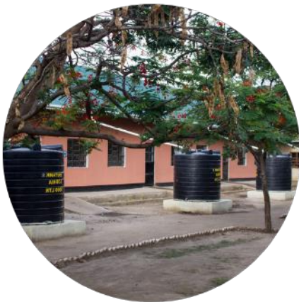
The community helped install the tanks for their local schools
